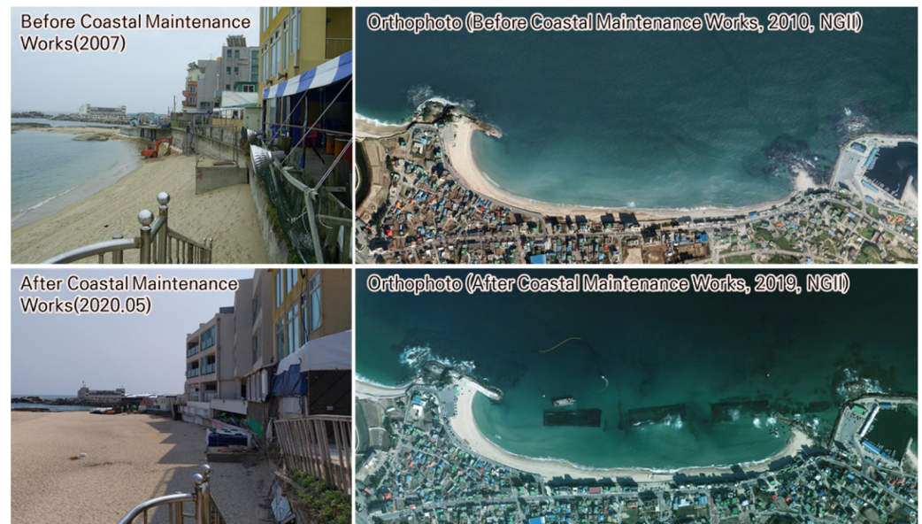
Figure 2. Before and after coastal maintenance work.
