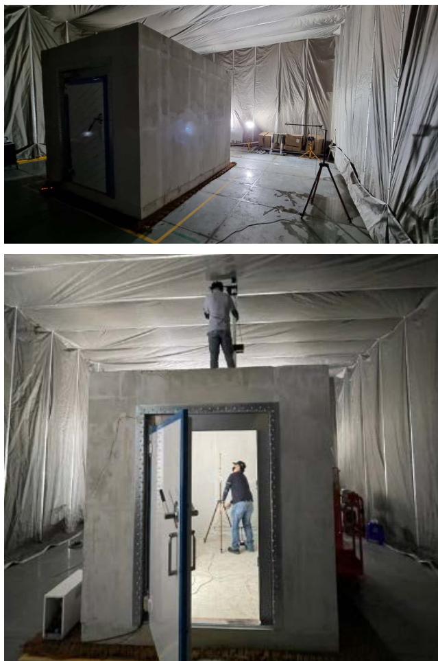
FIGURE 25. Concrete structure showing the shielding door in the rear side of the concrete structure that forms the SE test environment.
