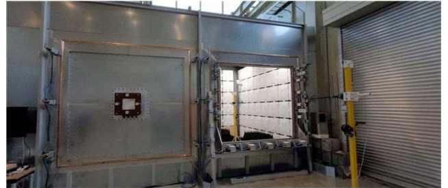
FIGURE 23. Construction of the anechoic room for testing the concrete wall.
