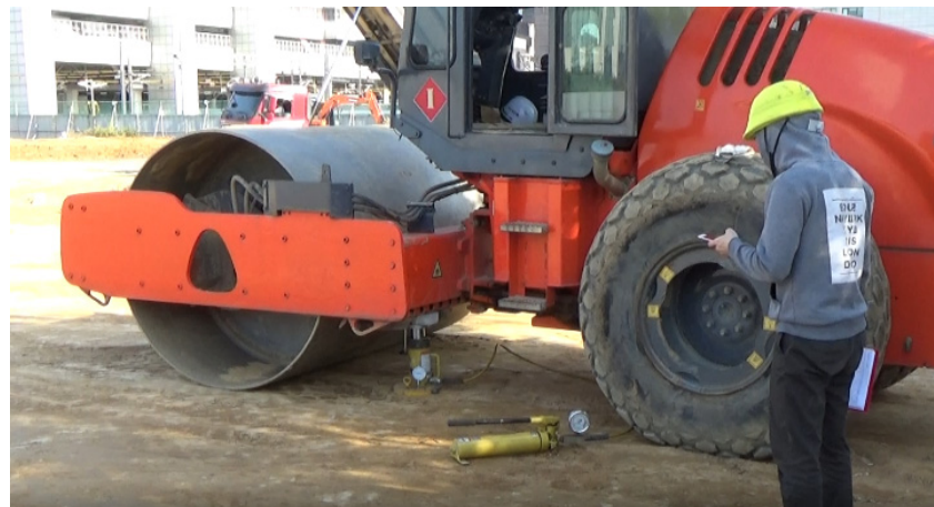
Figure 7. Plate load test arrangement at the construction site.
