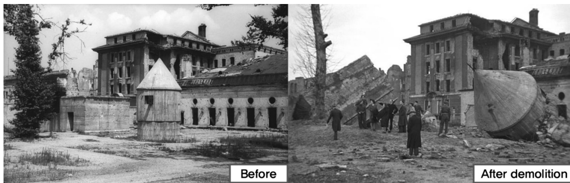
Figure 2. The demolished Führerbunker in the garden of the razed Reich Chancellery, Berlin (Bundesarchiv, Bild 183-V04744/CC-BY-SA 3.0; Bundesarchiv, Bild 183-M1204-319/CC-BY-SA 3.0).
