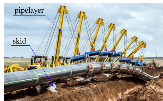
Figure 2. Pipeline during lowering-in [21].
